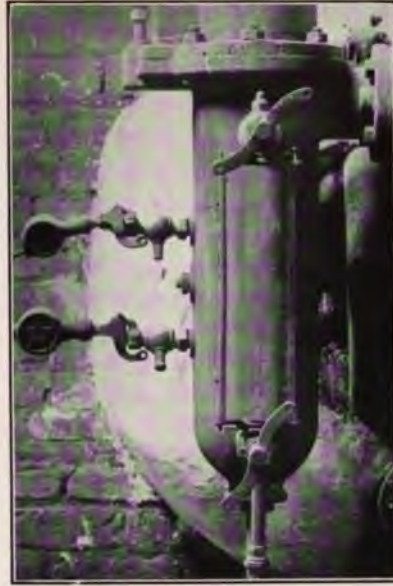
PLATES 3 AND 4.—GAUGE GLASS FOR INDICATING HEIGHT OF WATER IN A BOILER
